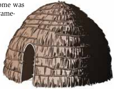
Twenty to 30 poles, about a foot apart, and bundles of grass were used to build a wickiup.
