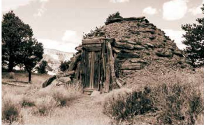
A Navajo hogan made of logs, small branches, brush, cedar bark, and earth
