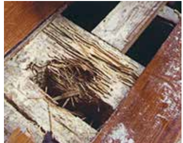
Termite damage
