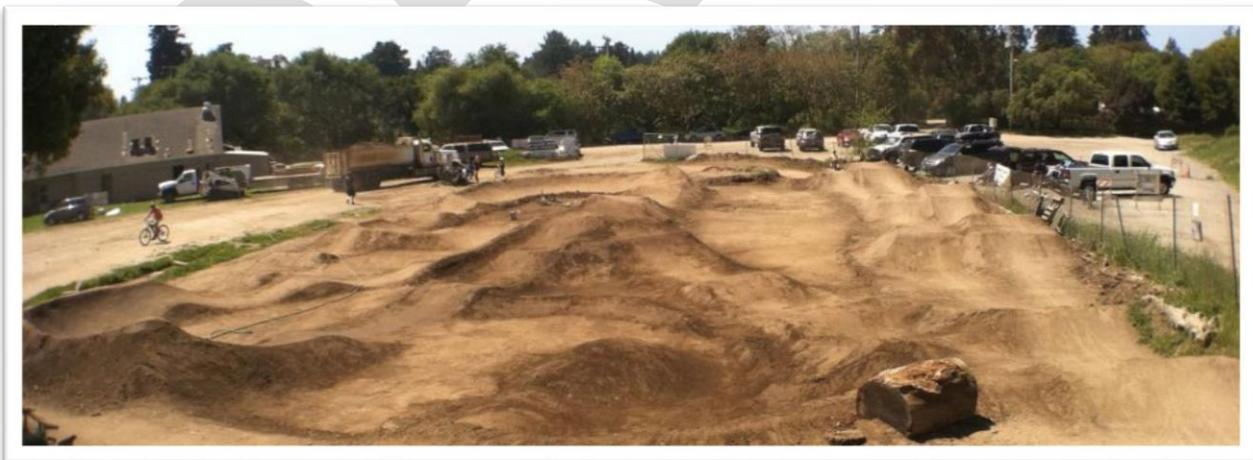
A 40 x 30—foot area takes 27 cubic yards. Pile dirt 50 percent higher than the final dimension to account for compaction. Then carve out the contours. "It's almost impossible to get a nice shape by adding dirt. It's easier to move it."
