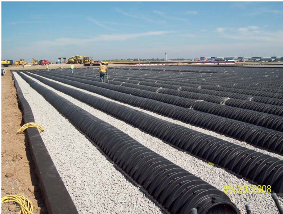
Figure 8 – Recirculating Gravel Filter under Construction
