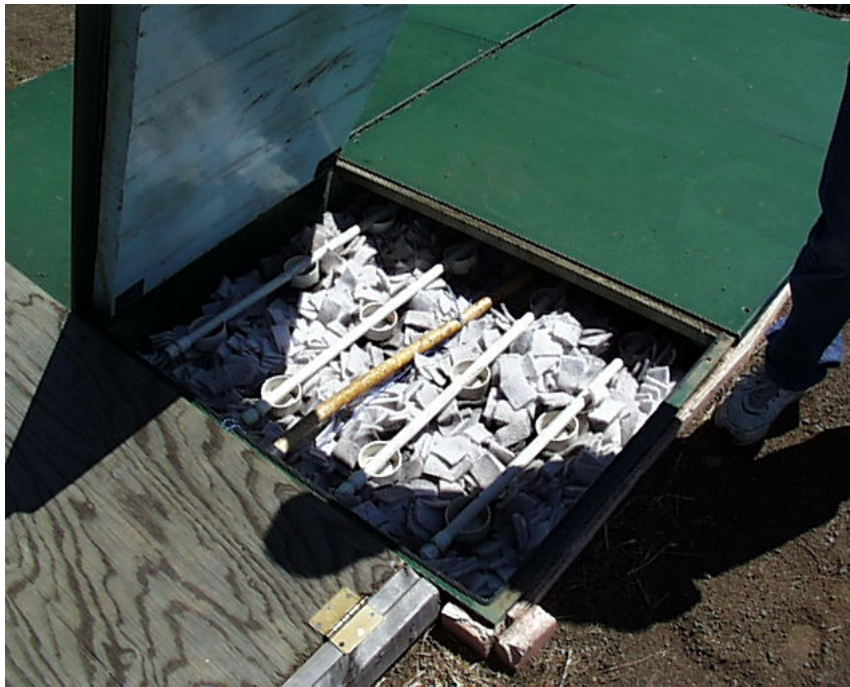
Figure 7 – Intermittent Filter using Cloth Media, Duluth Minnesota
