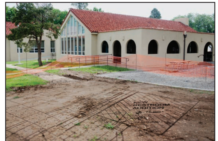
Construction is underway on new facilities at PTC. Josh Galemore/PhilNews
