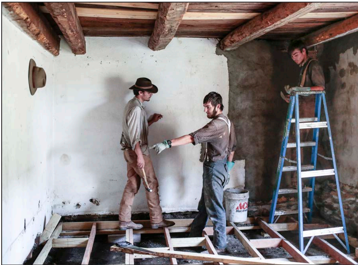
Inside the restoration room at Rich Cabins, foreman Peter Bergene and Adam Makin discuss what needs to be addressed as Cody Boruff applies plaster to a section of the wall on August 6, 2015. The Cabin Restoration team, which worked on the historic cabin for the past ten years, has restored flooring, walls and other aspects of the structure including installing a foundation beneath the standing house.
